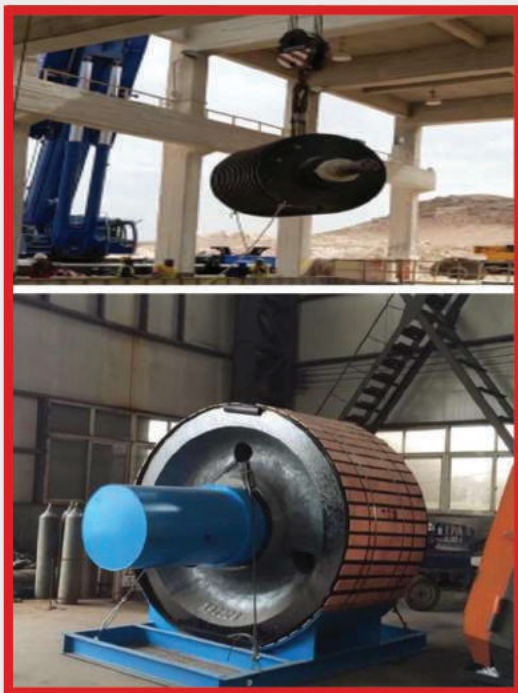
FLAP GAT DESIGN AND ERECTING MBCC
