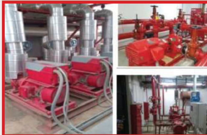
SUPPLING & INSTALLING FM200 & SYSTEM
